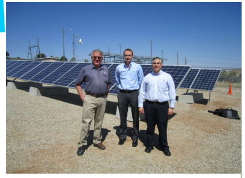
Cortez, CO (solar array owned by Empire Electric)
